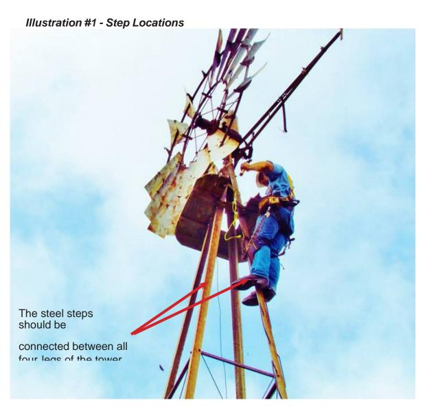
Installation of steel steps should be below the level of the work platform at all aspects of the tower. These steps provide placement for a technician to stand on while connecting a chain between the outer band of the fan wheel and the upper tower during the tower head lock off procedure.
