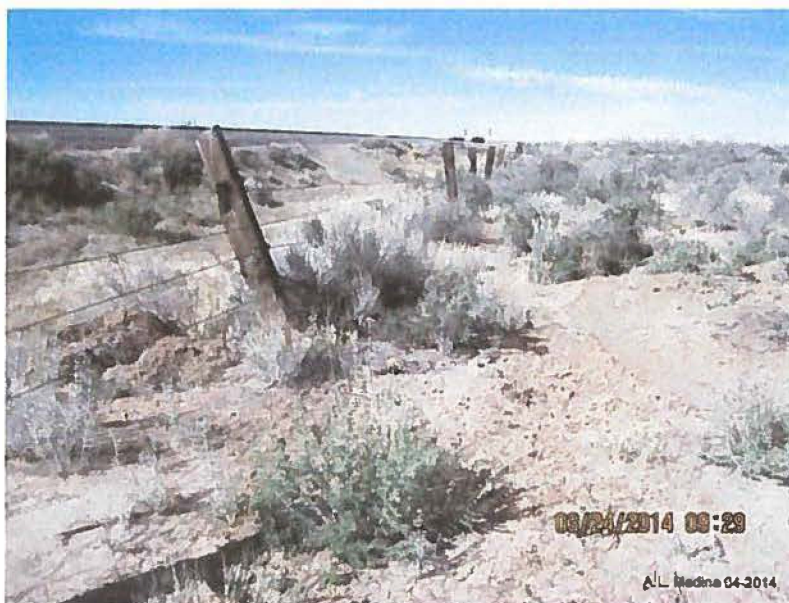
Figure 10. This photo shows a historical fence where railroad ties were used as line posts. These are rare on New Lands.
