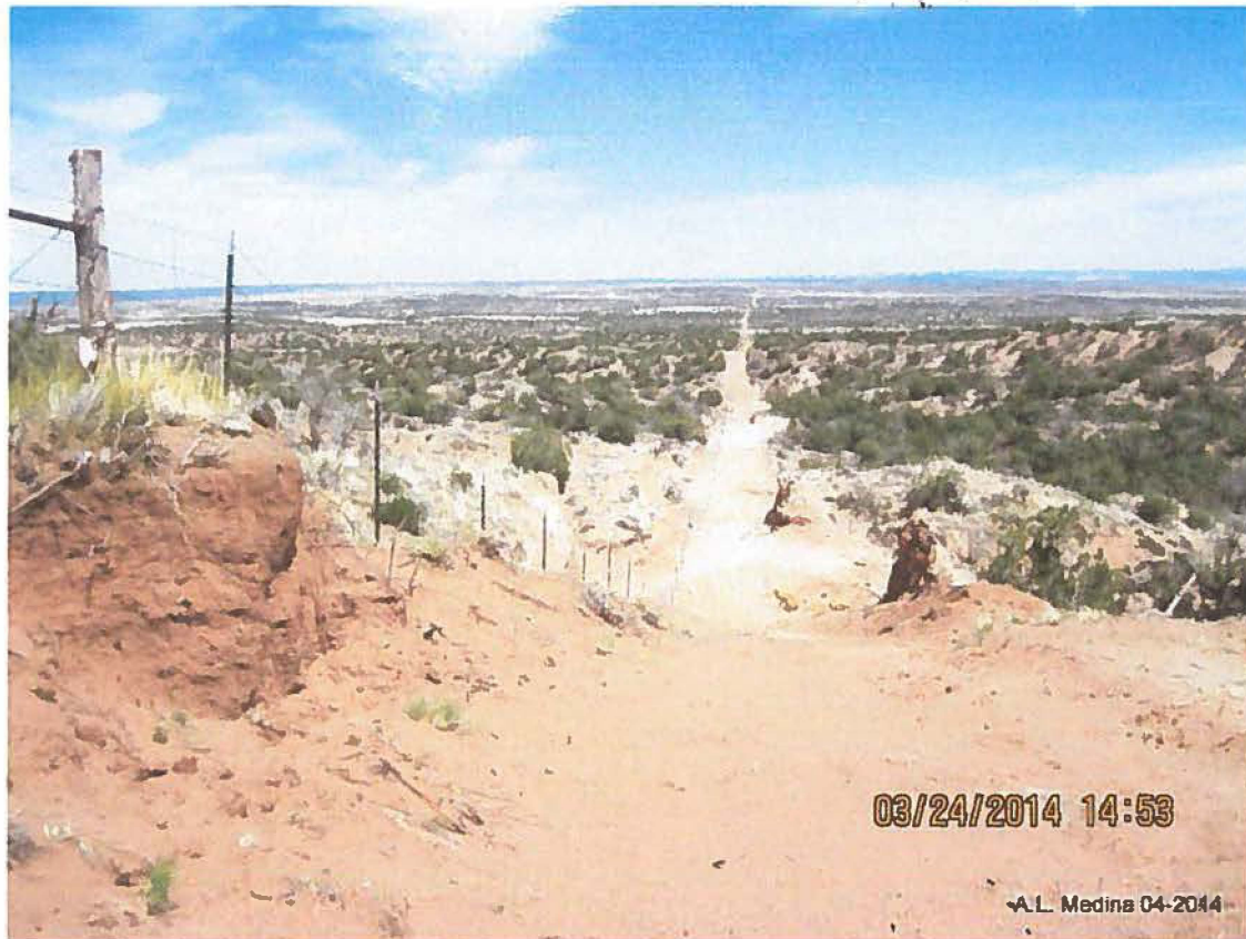
Figure 9. This photo shows the bladed area where the fence was realigned. The action resulted in several areas where the blade made too close contact with the fence and compromised their footing.
